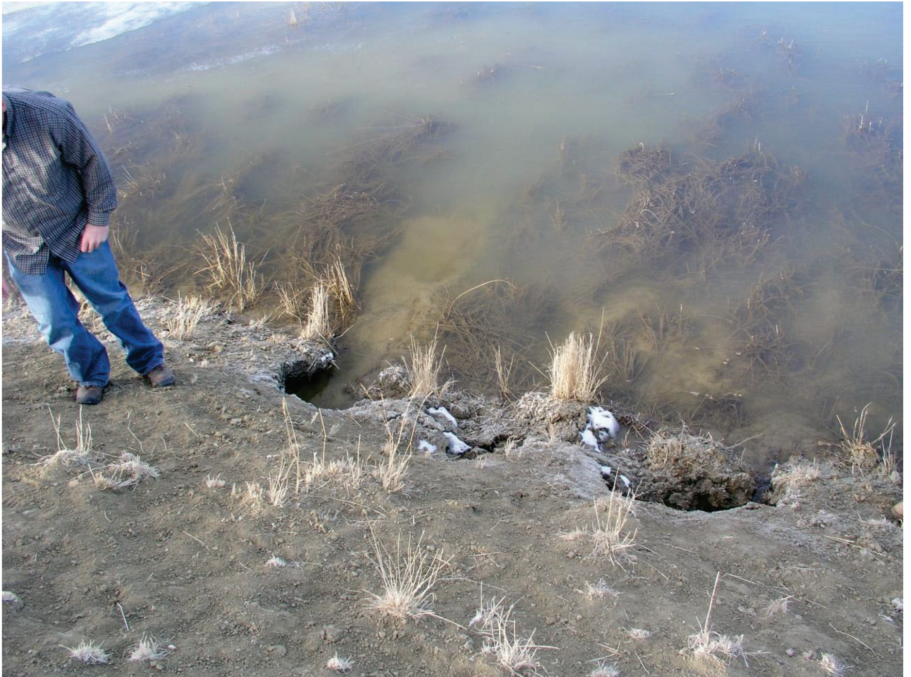
Picture 4 - Sloughed Material
